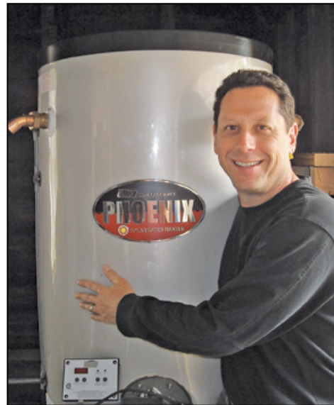
David Gottfried with his new Phoenix Solar unit: "It is neat to showcase our ability to generate domestic hot water and space heating from a single tank."
